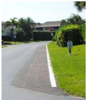
The walkway along Windward Drive is nearly complete. The asphalt has been laid. All that remains is the striping which should be completed by the end of the month. As a part of the project, all of our roadways will be restriped and markings (like Stop) will be restenciled.
